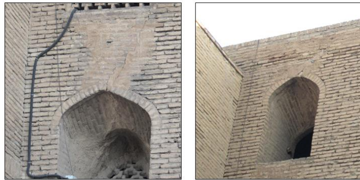
Fig 3 and 4 Cracks on the northern side of the mosque wall
