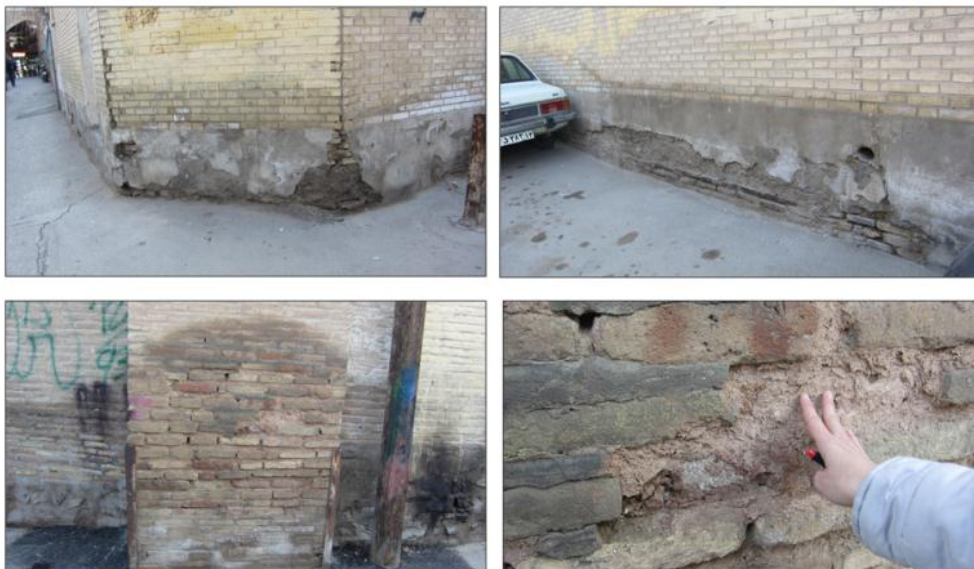
Photo 5 to 8 Caries, corrosion and moisture in buildings in the sides of mosque's adjacent streets
