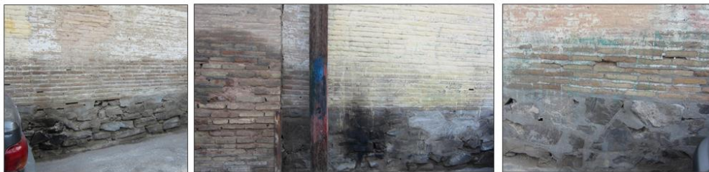
Photo 11 and 13 Use of stone and cement sand mortar in the perimeter wall of the mosque
